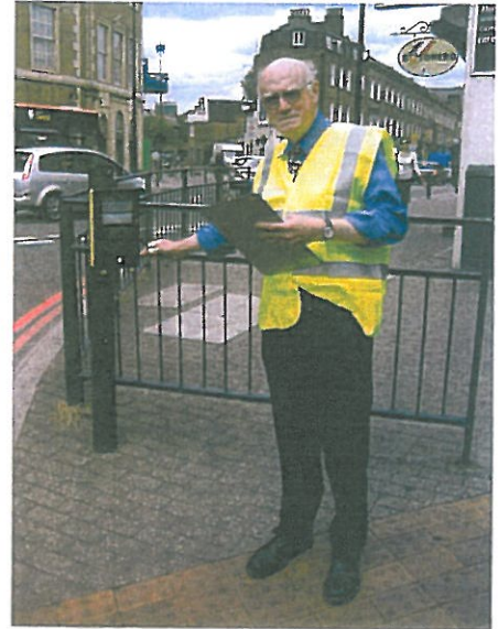
A blind or partially sighted pedestrian standing on the tactile paving wouldn't be able to reach the pedestrian push button facility
