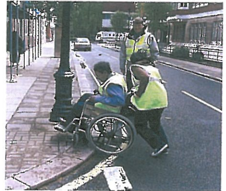
Even a modest kerb upstand can present a barrier to a wheelchair user, TMS Consultancy's Mark Steventon points out
