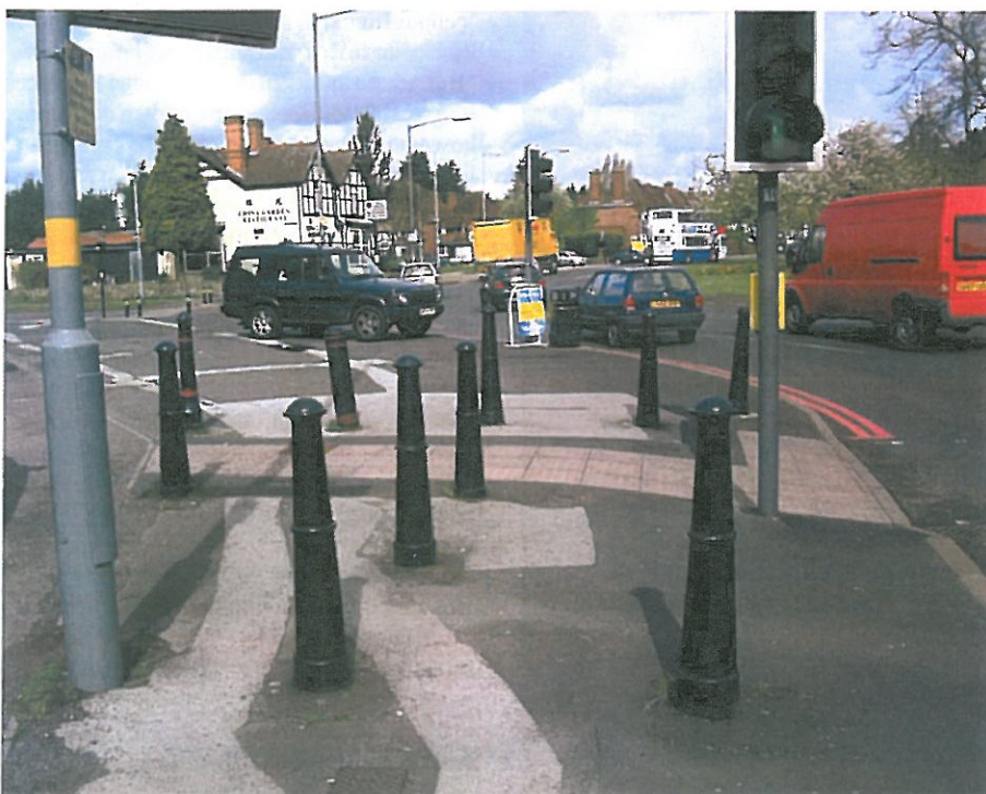
A maze of redundant bollards create an obstacle course near to a crossing
