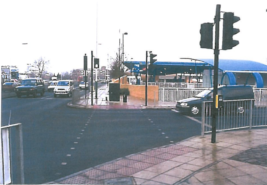
The alignment of the tactile paving should guide a blind person safely across to the other side: in this case, however, it misdirects a pedestrian towards traffic on the main road
