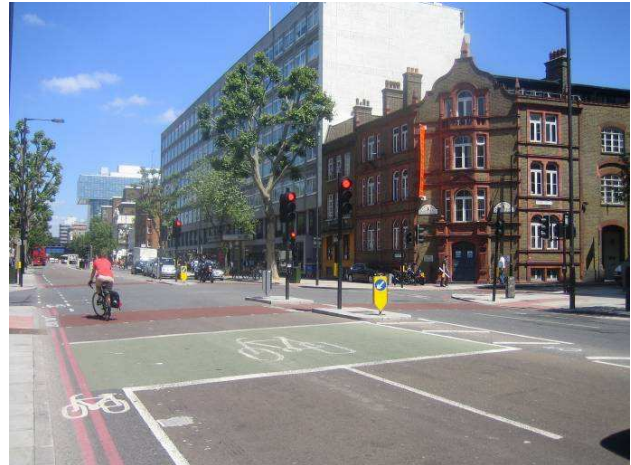
Another Borough, where a signal junction has been re-modelled with no guardrail
