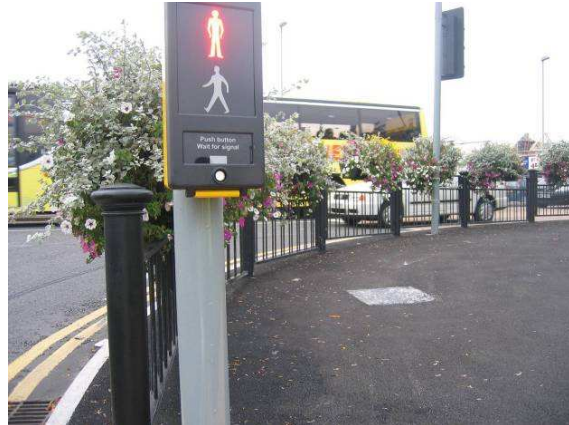
Attempts to make guardrail less unsightly have led to a different potential safety problem
